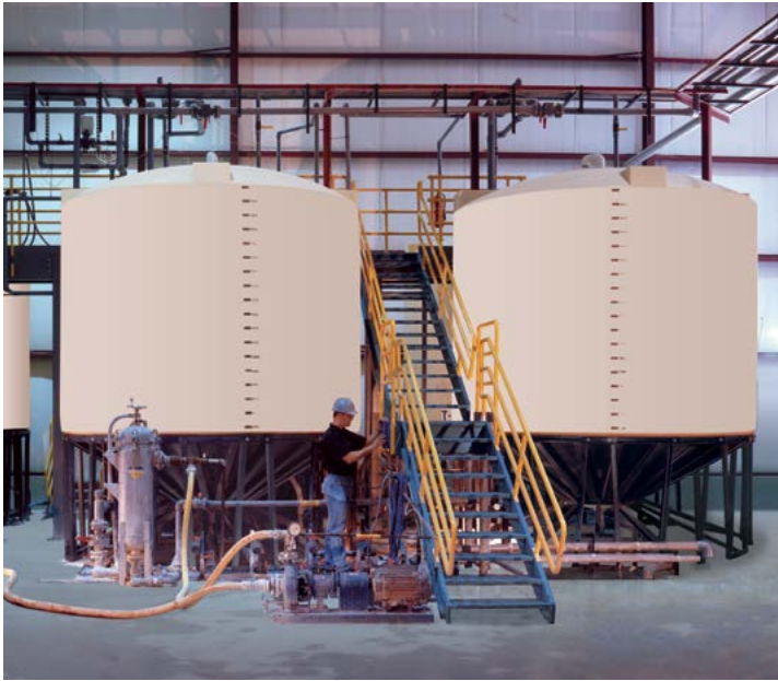
Assmann conical bottom storage tanks at a central Indiana chemical company.
