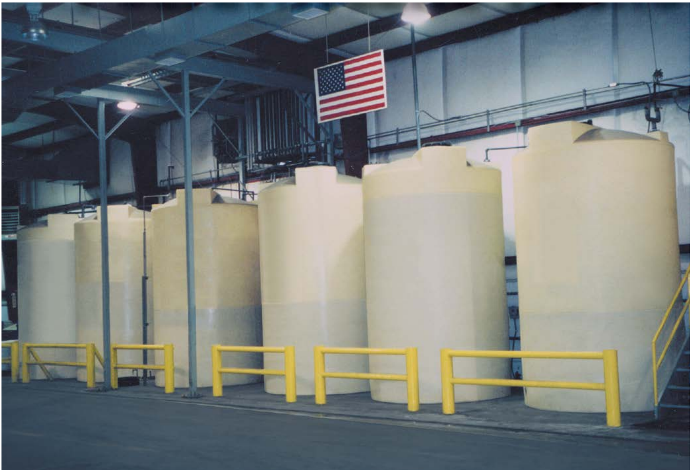
Chemical storage facility located in Virginia.
